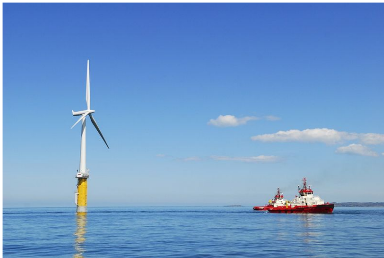
Figure 5: Hywind tugged to location outside Karmøy
