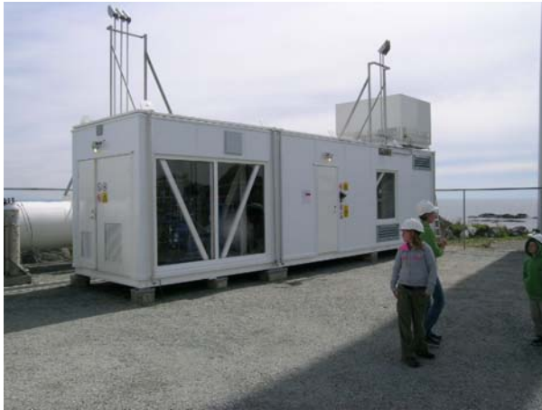
Source: Electrolyser in front and storage vessel behind (Eide et al. 2004)
